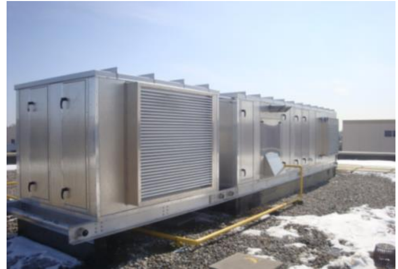
Gas-fired make-up air vents
