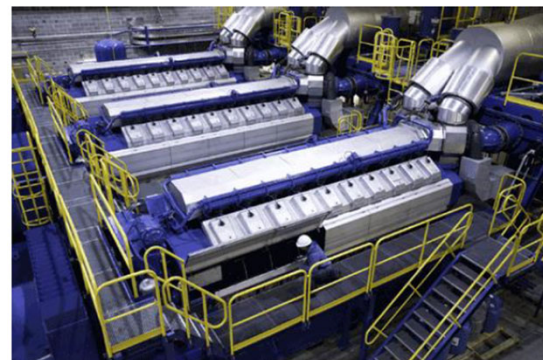
Reciprocating Engine Power Plant (source: Wartsila)
